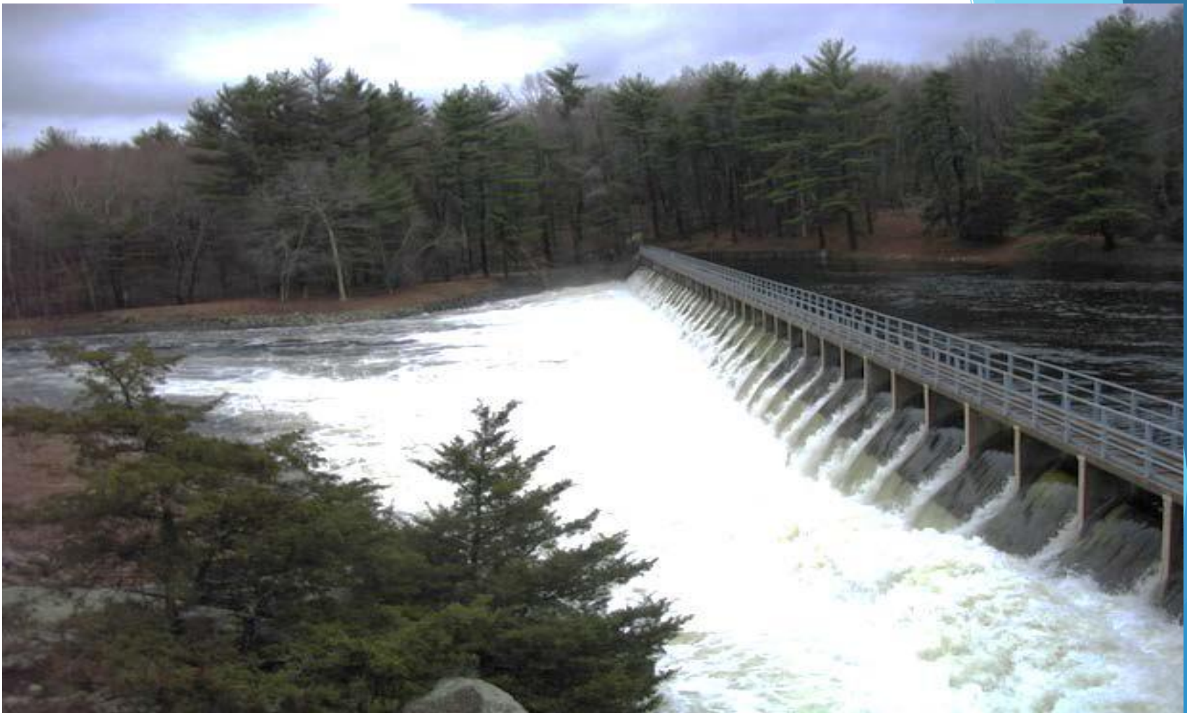
Figure 3: The Gainer Dam spillway at the Scituate Reservoir at 10:30 a.m., March 31st, 2010. Flow was an unprecedented 2.5 feet over the flashboards at a pool elevation of 287.80 feet. See Figure 2 for the spillway on a normal day, with only a trickle flowing over the flashboards. (David Vallee, National Weather Service Northeast River Forecast Center (NWS/NERFC))
